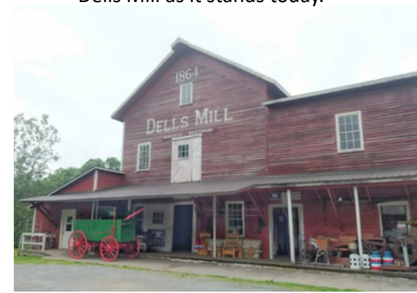
Dells Mill as it stands today.
